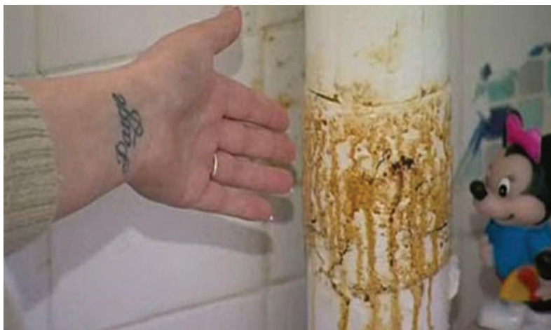
FIGURE 3.2 Living in substandard conditions: sewage invasions in Dolphin House local authority estate, Dublin's inner city (photograph by authors)
